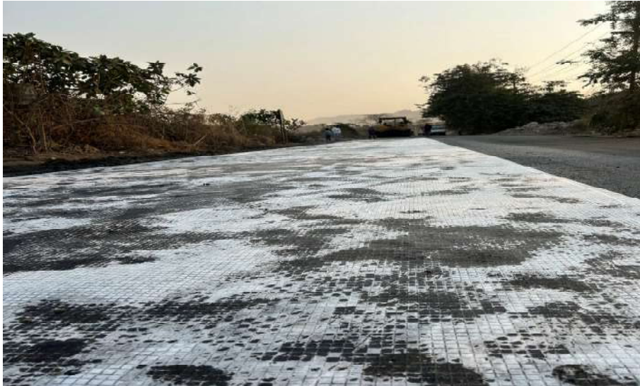
Geogrid Reinforced Asphalt pavement Trial section – Navi Mumbai
