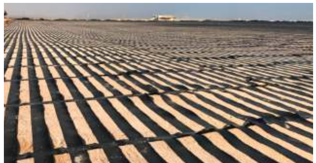
ParaLink® used in basal platform, Mexico
